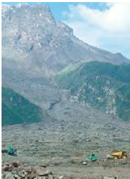
Fig. 3. Multiple cooperating construction robots are operated by a single human supervisor from a central box, Vision Sketch Japanese Research Institute, 1980
