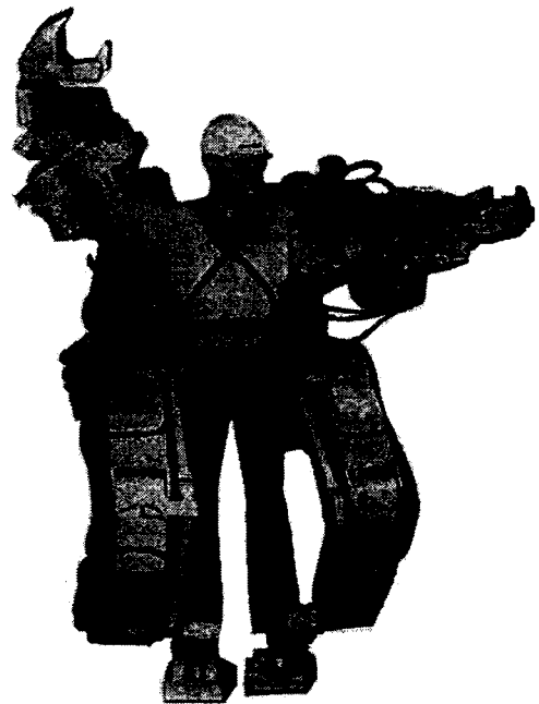
Fig. 3-1 "Hardiman" exoskeleton built by G.E. in the 1960's [42].
